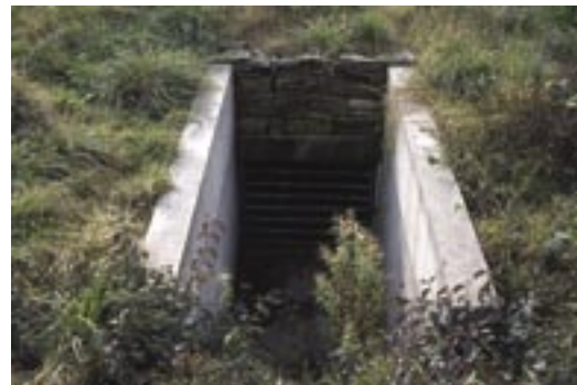
Small grilled mine in sloping ground, UK.
