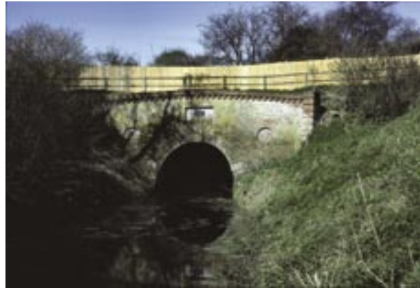
Greywell canal tunnel grille.
