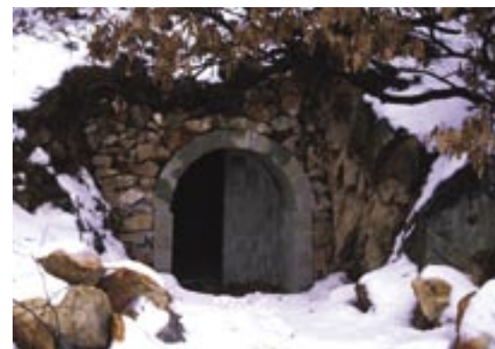
Király-bányák mine entrance after reconstruction and improvement.
